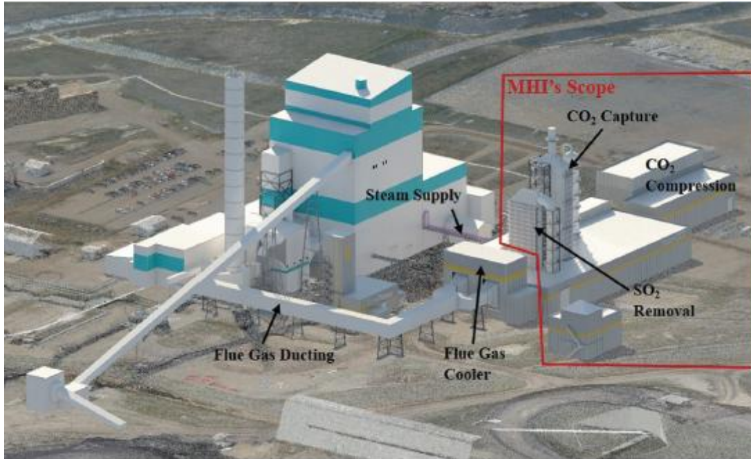
Figure 4-7. 3D Depiction of Shand Unit 1 Equipped with CCUS Process Equipment
