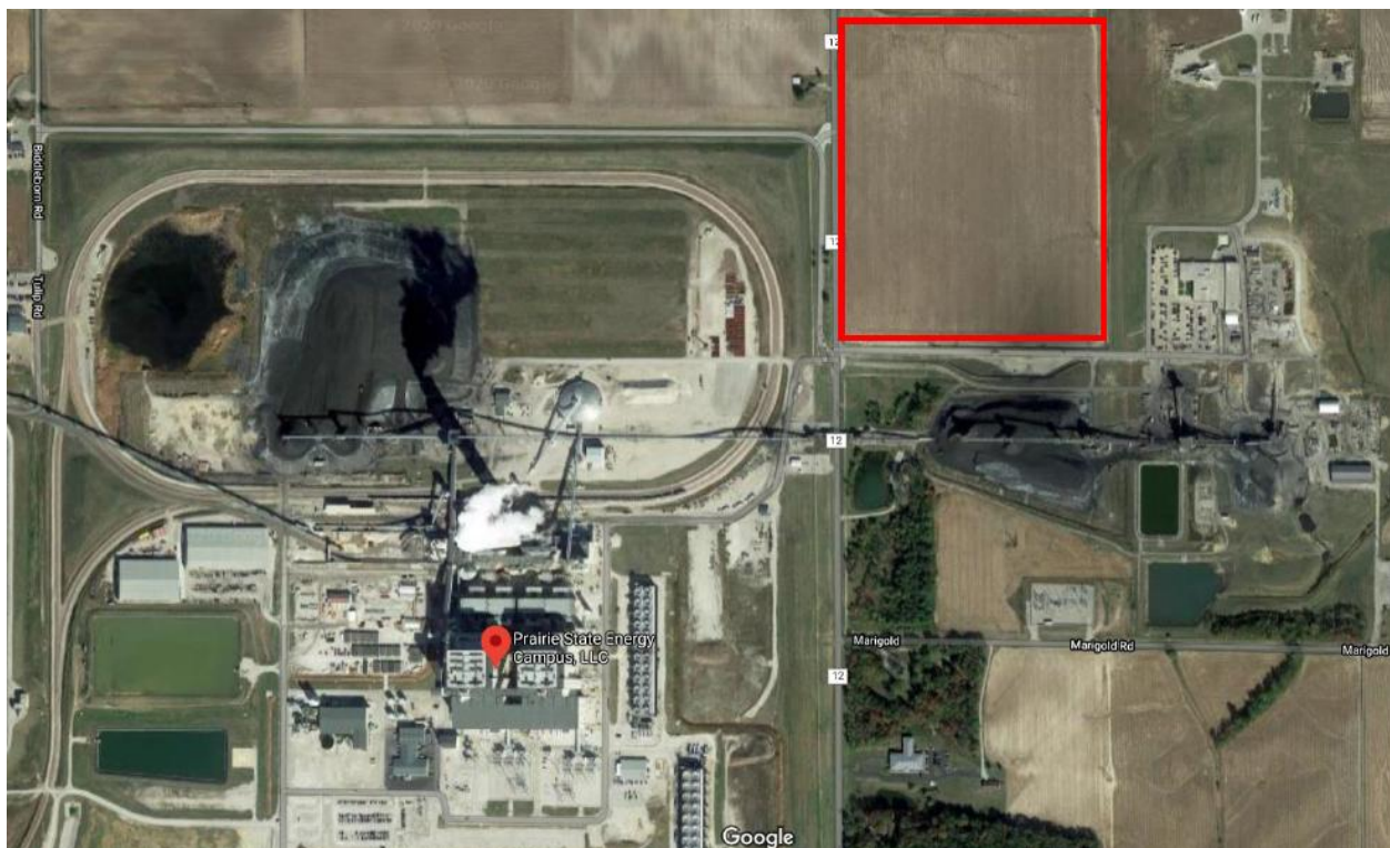
Figure 4-6. Prairie State Generating Station Unit 2 with Footprint for CO 2 Capture Island
